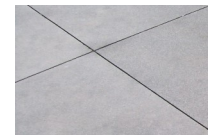
Cut and Grout
